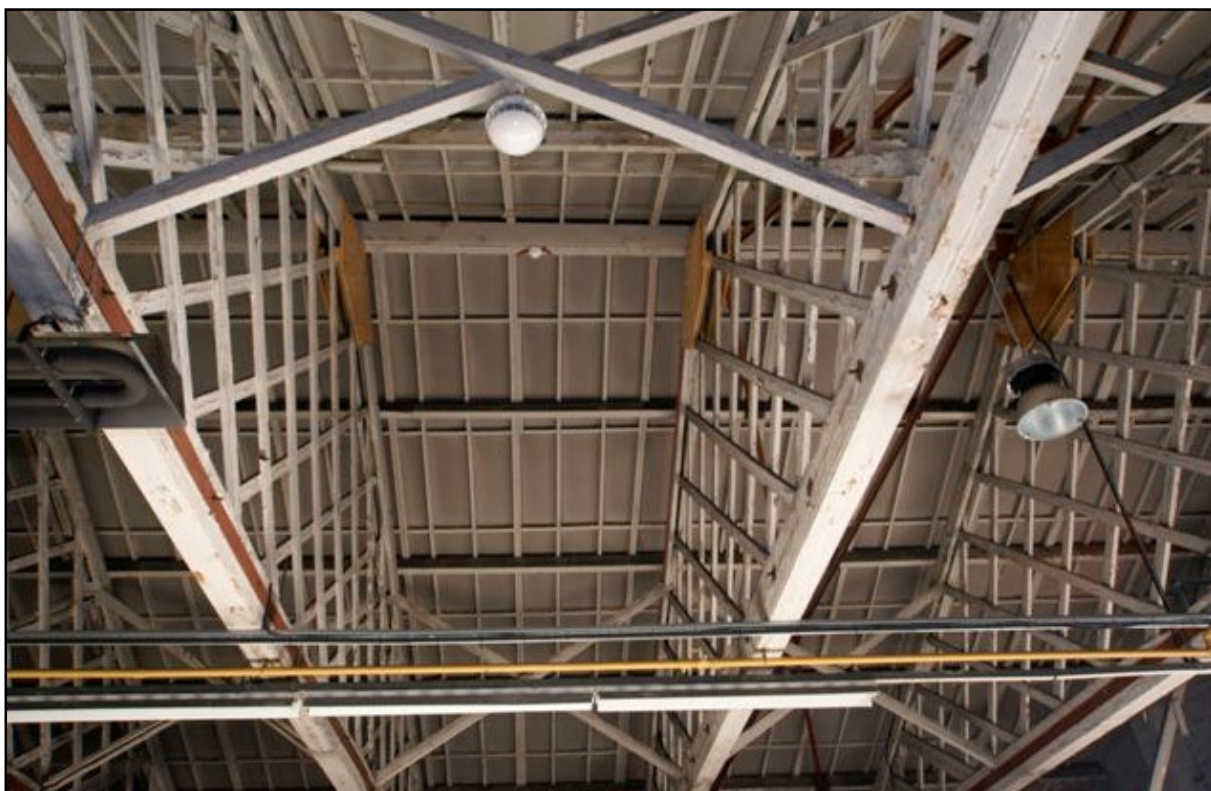
Plate 8: Shed 1, Bay 'A' – interior view of trusses and wind bracing struts
